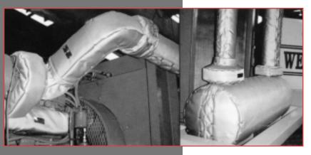
Ceramic Fiber blanket and a woven Fiberglass Impregnated with Silicone Resins. The blanket is firmly stitched with Kevlar thread and is reusable. It resists damage, absorbs sound and is suitable for operating temperatures up to 1000 degrees Fahrenheit. If TIB becomes wet, from water, steam, or oil, its thermal and physical properties are restored after drying. Our TIB also meets the U.S.
